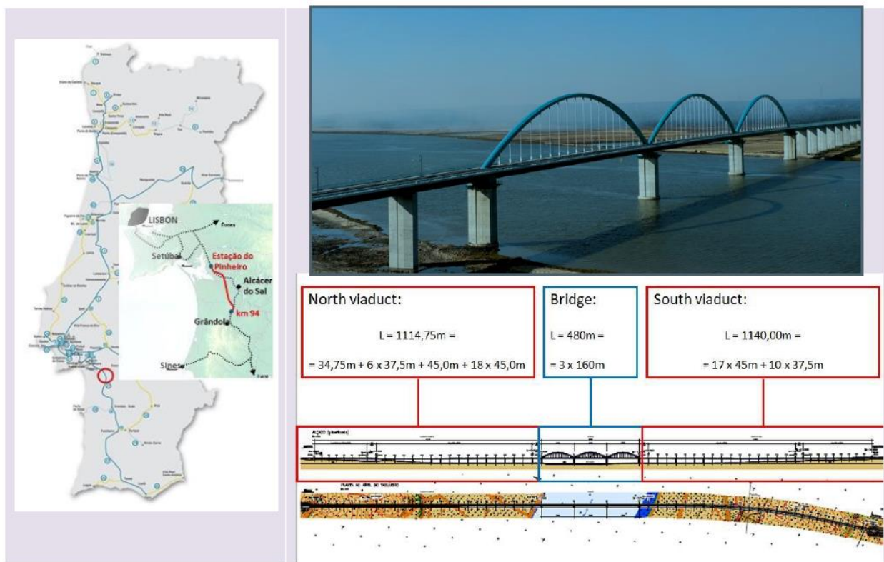
FIGURE 5. LOCATION AND GENERAL VIEW OF THE RAILWAY BRIDGE OF ALCÁCER DO SAL
