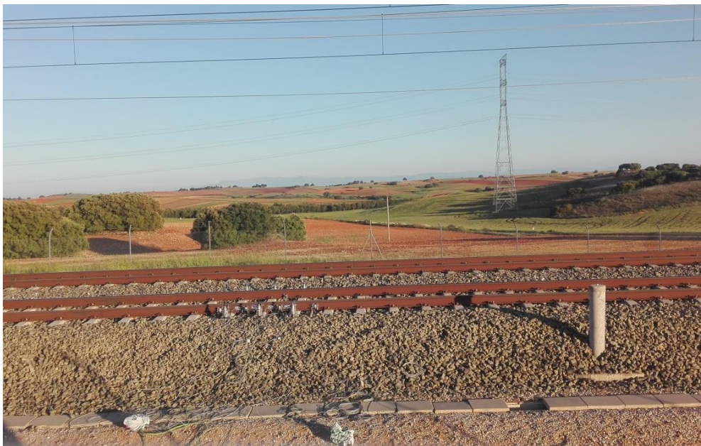
FIGURE 35: PK 74+233 MADRID-BARCELONA HIGH SPEED LINE- STRAIGHT TRACK SECTION
