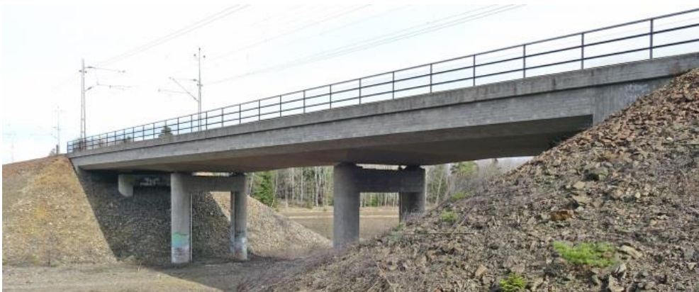
FIGURE 41. THE BEAM BRIDGE AT PERSHAGEN.
