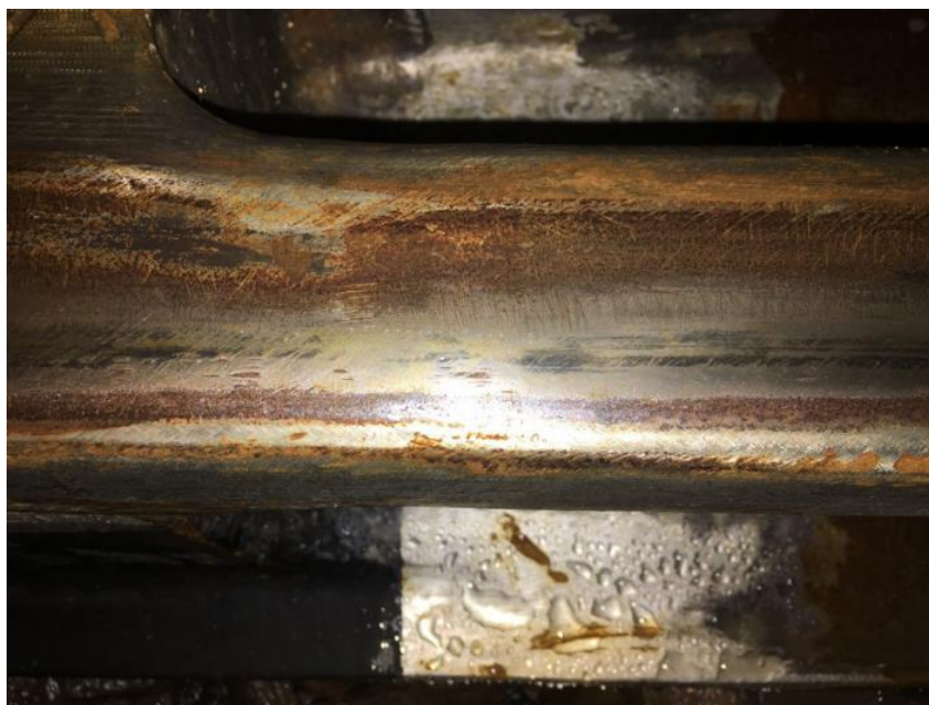
FIGURE 29. DETAIL OF THE RUNNING SURFACE OVER WELD A – DIRECT LINE
