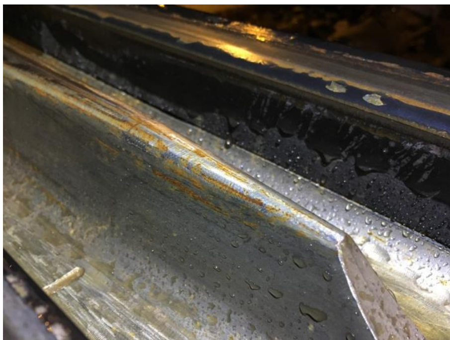
FIGURE 28. DETAIL OF THE CROSSING NOSE
