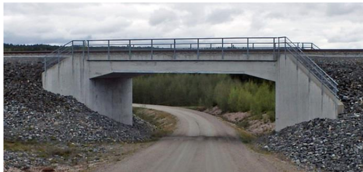
FIGURE 38. THE PORTAL FRAME BRIDGE AT ORRVIK.
