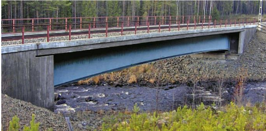
FIGURE 39. THE PORTAL FRAME BRIDGE AT SKIDTRÄSK
