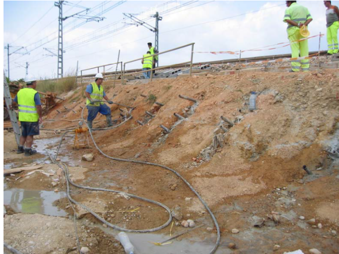
Figure 4.1.29. grouting operations (European Project SUPERTRACK, 2005)
