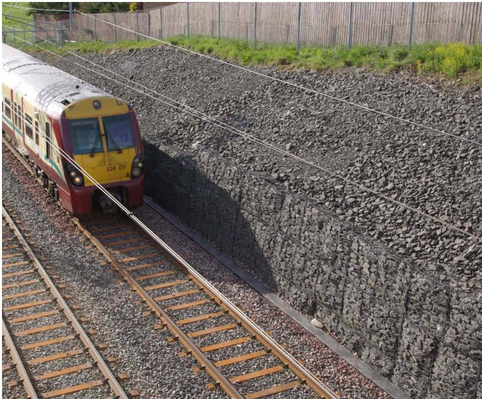
Figure 4.2.34. Gabion retaining wall at the new Airdrie to Bathgate passenger rail link in the central belt of Scotland is a landmark project by Network Rail to widen and re-open a 24km line closed over 50 years ago. Gabion (2015).
