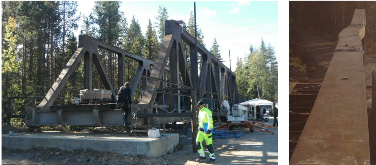
Figure 4.2.8. Test of 55 year old 33 m long metallic bridge at Åby River in 2013. Overview of test site with two jacks anchored in the bed rock in the centre (left) and final buckling failure of top girder beam (right), ML-D1.3 (2015).
