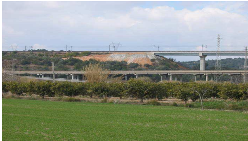
Figure 4.1.28. general view of the embankment where the soil improvement was achieved (European Project SUPERTRACK, 2005)
