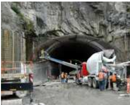
Figure 4.2.27. The Weehawken Tunnel in New York was in 2006 widened from 8.4 x 6.4 m to 19.7 x 10.4 m, see Berliner et al (2004). Photos by John Papas 2004 and David Pirman 2006.
