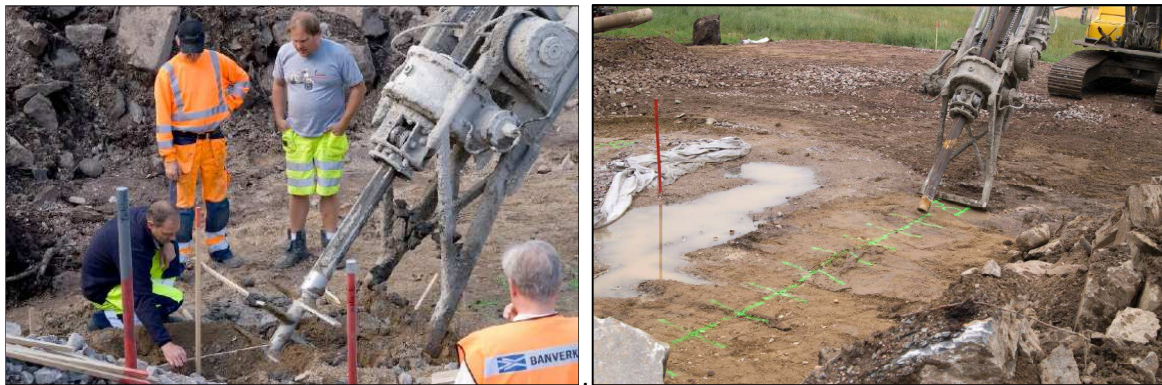
Figure 2.1.19 Positioning of lime cement columns
