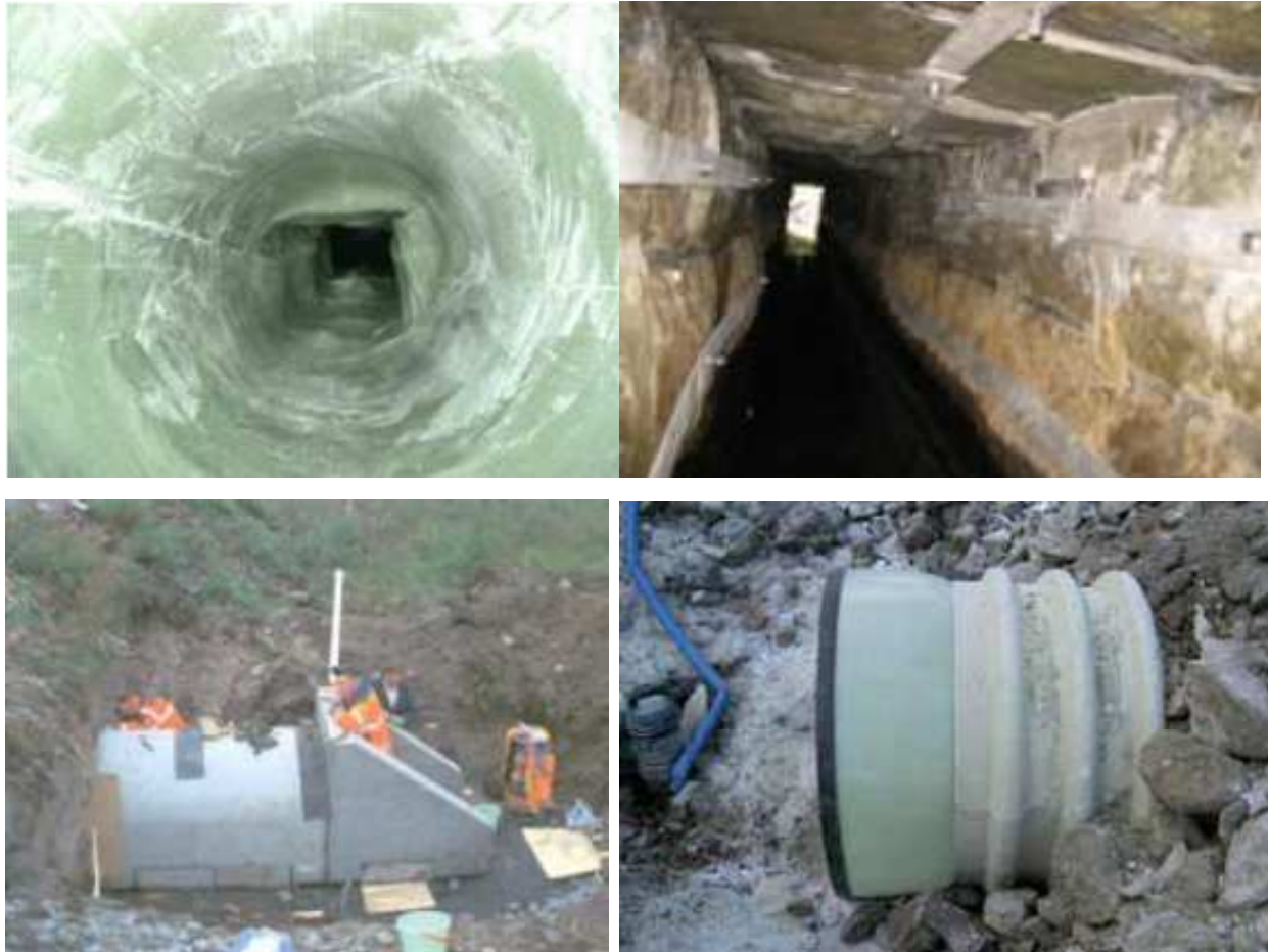
Figure 4.2.31. Examples of measures to restore culverts (from top left clockwise): (a) Lining with plastic material; (b) Repair of joints; (c) Extension of culvert; (d) Corrugated steel culvert repaired with glass fibre lining. The lining expands at the ends of the culvert and stabilizes the embankment. Södergren (2011), Railcare (2012), ML-D1.1 (2013).
