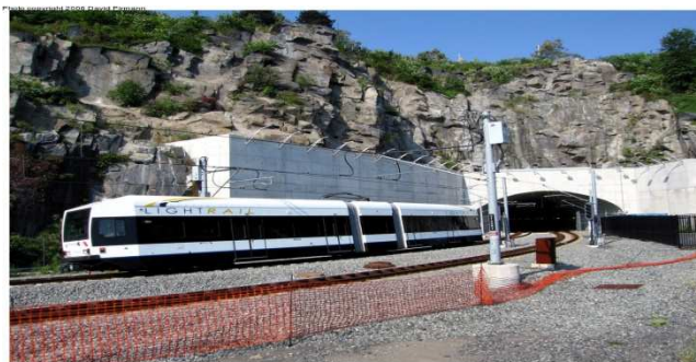
Figure 4.2.27. The Weehawken Tunnel in New York was in 2006 widened from 8.4 x 6.4 m to 19.7 x 10.4 m, see Berliner et al (2004). Photos by John Papas 2004 and David Pirman 2006.
