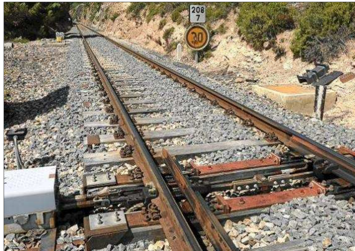
Figure 4.1.30 Treated railway section (Escudero, 2011)
