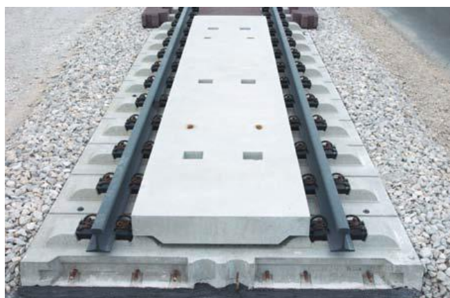
Figure 34. FF Bögl slab track system. Derailment protection device.
