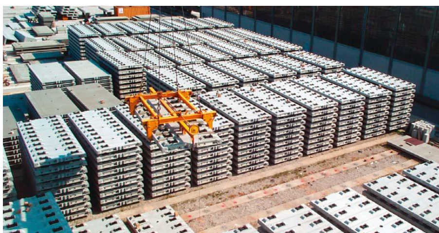
Figure 23. Storage of FF Bögl precast slabs [40]
