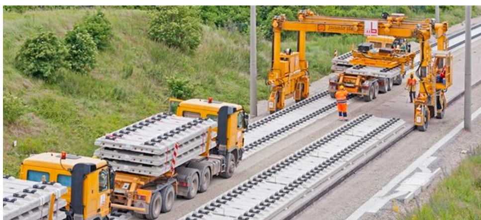
Figure 26. Transportation and rough placing of precast slabs [40]
