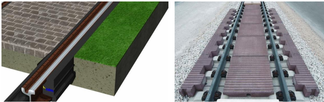
Figure 19. Left: Artificial Grass Track, CDM [26]. Right: Absorbing elements, FF Bögl [10].
