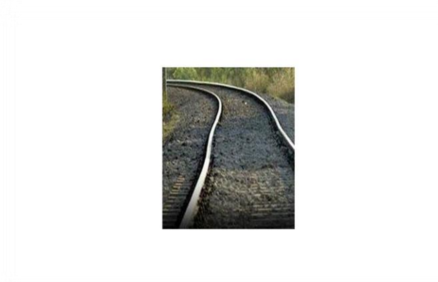
Figure 4.2.1. Failure of track geometry due to warm weather
