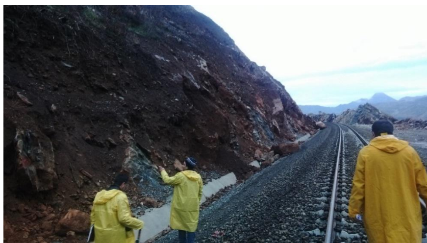
Figure 4.3.3. Fallen rocks due to rain
