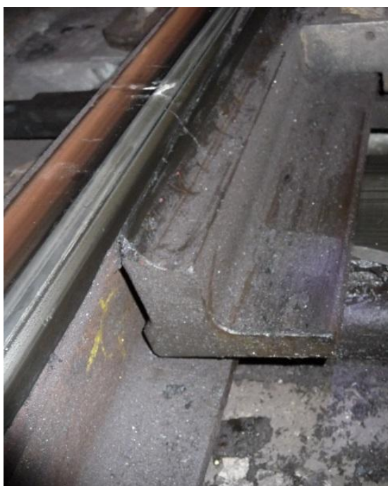
Figure 3.1.3. View of coupled switch rail and stock rail (allowing for diverging track)
