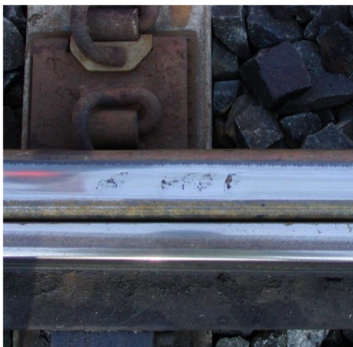
Figure 3.1.1. Wear on the switch rail and RCF on the stock rail caused by high tangential contact stresses. From [3.1.2]
