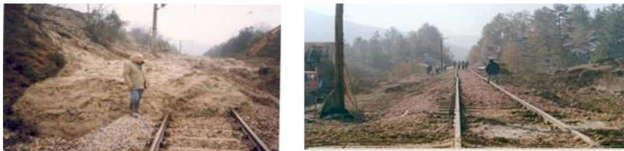
Figure 4.3.1. Landslide due to extreme rain
