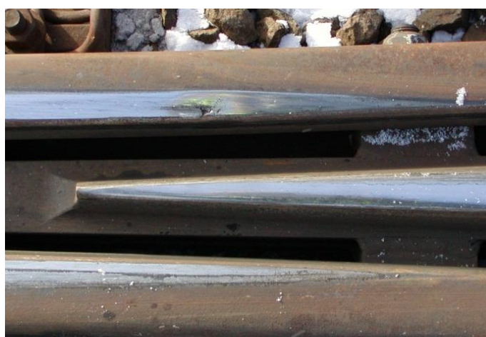
Figure 3.2.5. Example damage of wing rail – plastic deformation and localised crushing in contact area
