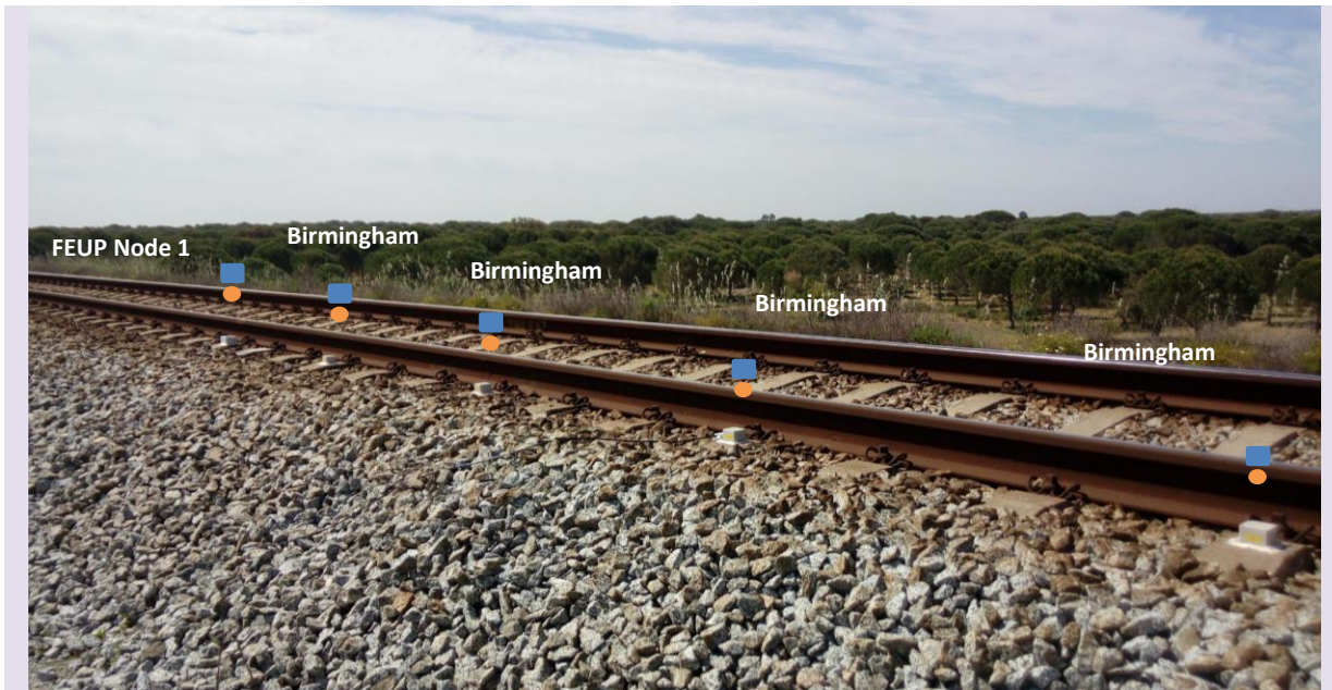
FIGURE 27 – SENSORS DISTRIBUTED IN THE TRANSITION
