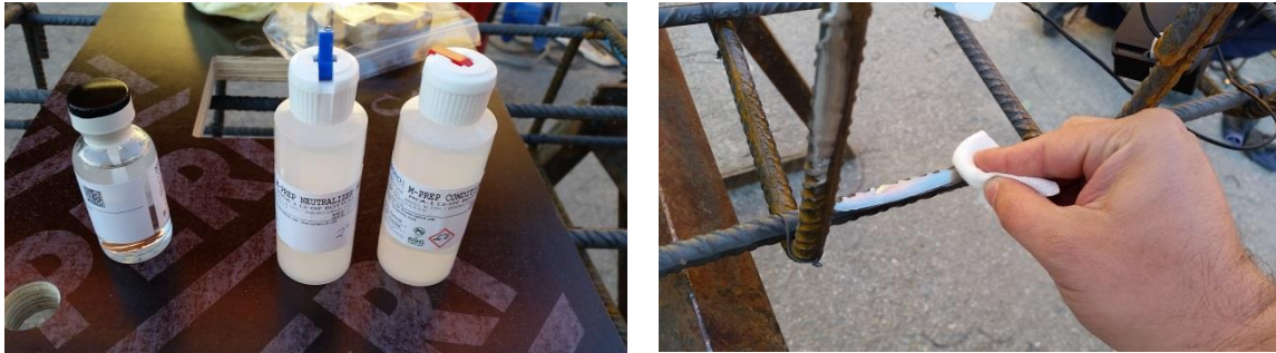
FIGURE 7. CLEANING THE SURFACE OF THE BARS THROUGH THE USE OF AN ACID AND BASIC SOLUTIONS
