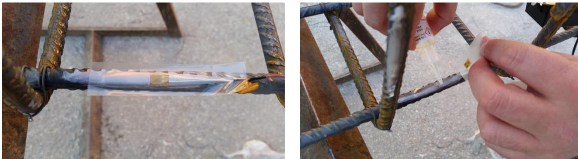
FIGURE 8. GLUING OF THE STRAIN GAUGE IN THE BARS
