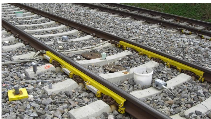
FIGURE 10 ADDITIONAL SENSORS TO MEASURE FORCES, ACCELERATIONS AND PORE WATER PREESURE AT THE CRITICAL SECTION
