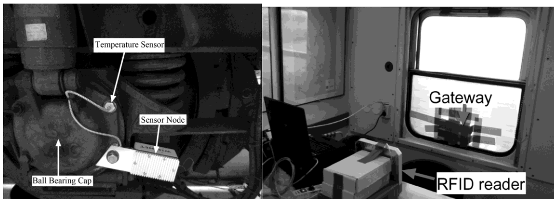
Figure 6.4: Left: One of the sensors mounted on the ball bearing cap. The electronics are located inside the white box and the temperature sensor is located inside the bolt. The cable from the sensor to the node is covered by metal. Right: The setup aboard the wagon with gateway (GW) and RFID reader.
