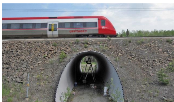
Figure 17. The soil-steel composite bridge at Märsta during passage of an X52 train, reproduced from [26].
