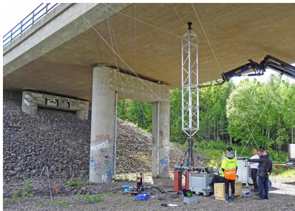
Figure 22. The beam bridge at Pershagen, during testing with the hydraulic exciter, [28]
