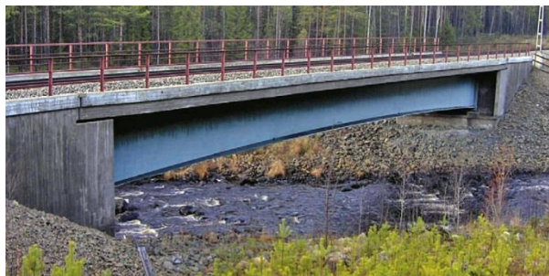
Figure 15. The portal frame bridge at Skidträsk, reproduced from [22].
