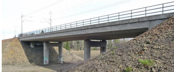
Figure 21. The beam bridge at Pershagen. [28]
