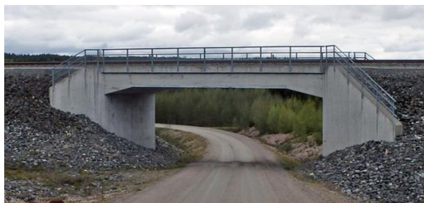
Figure 13. The portal frame bridge at Orrvik.
