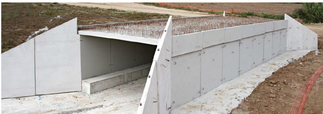
Figure 182. View of a similar bridge during construction, Forte (2010).
