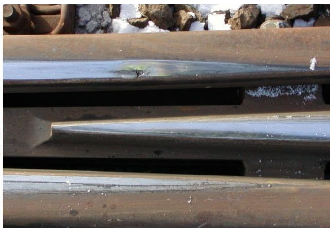
Figure 3.2.5 Example of damage on wing rail – plastic deformation and localised crushing in contact area. The damage is in the order of few 10s of mm, matching the definition of the P1 force.
