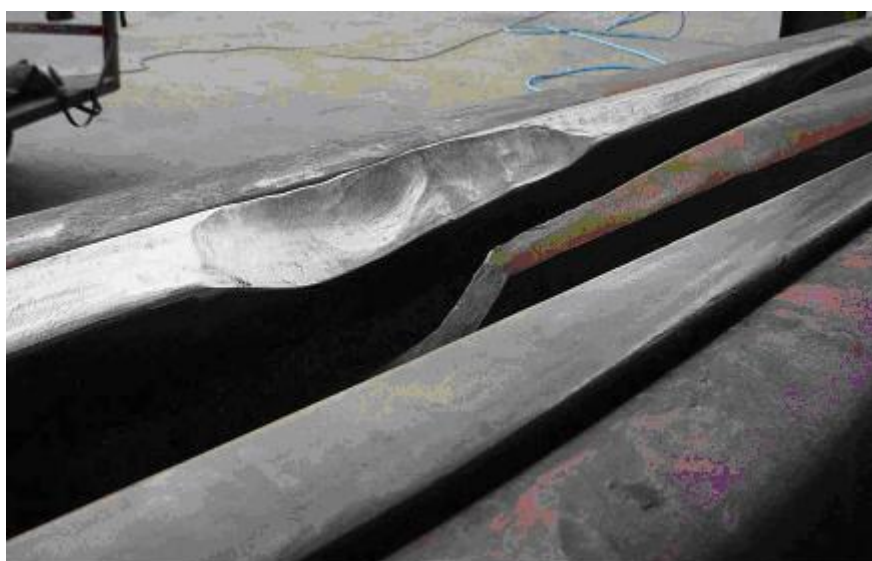
Figure 3.2.56 Example of the Extent of Weld Repairs Required [3.2.58]
