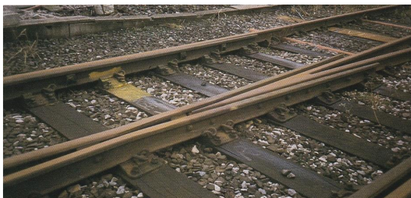
Figure 3.2.43 Part Fabricated Crossing [3.2.52]
