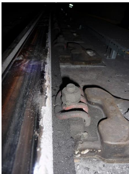
Figure 3.1.5 Stock rail on the right side. View of the field side seen from the switch toe
