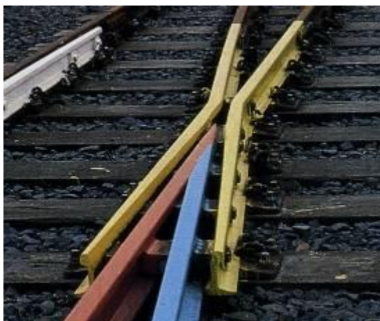
Figure 3.2.42 Fully Fabricated Crossing [3.2.52]
