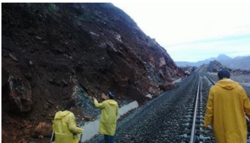
Figure 4.4.3 Fallen rocks due to rain
