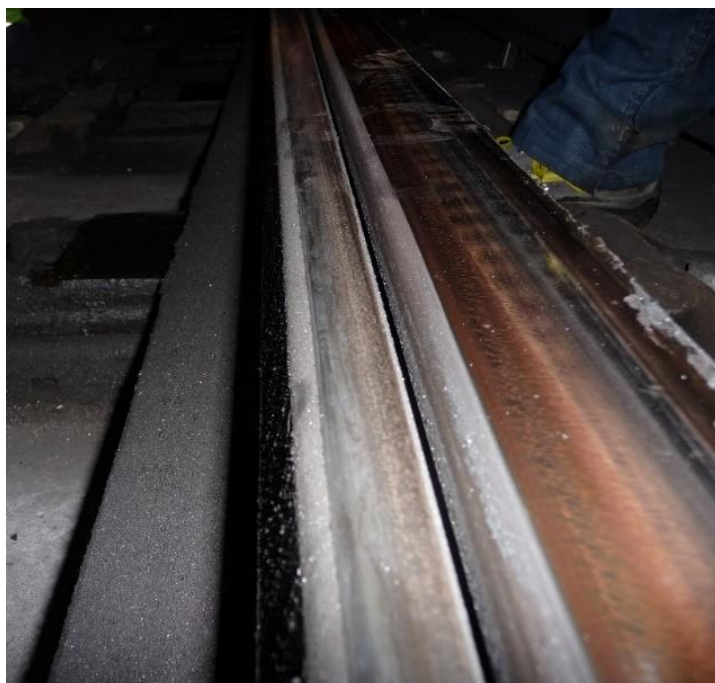
Figure 3.1.4 Stock rail on the right side. When uncoupled, it allows for traffic to diverging track
