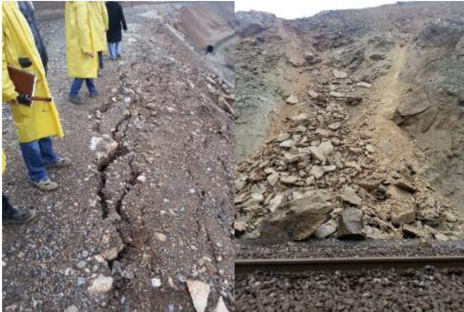
Figure 4.4.4 Landslide due to excessive rain (left) and unavailable track due to fallen rocks caused by excessive rain (right)
