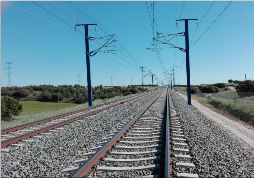
FIGURE 26: VIEW FROM THE TRACK. THE SECTION IS STRAIGHT IN SOME KILOMETERS BEFORE AND AFTER THE SELECTED POINT
