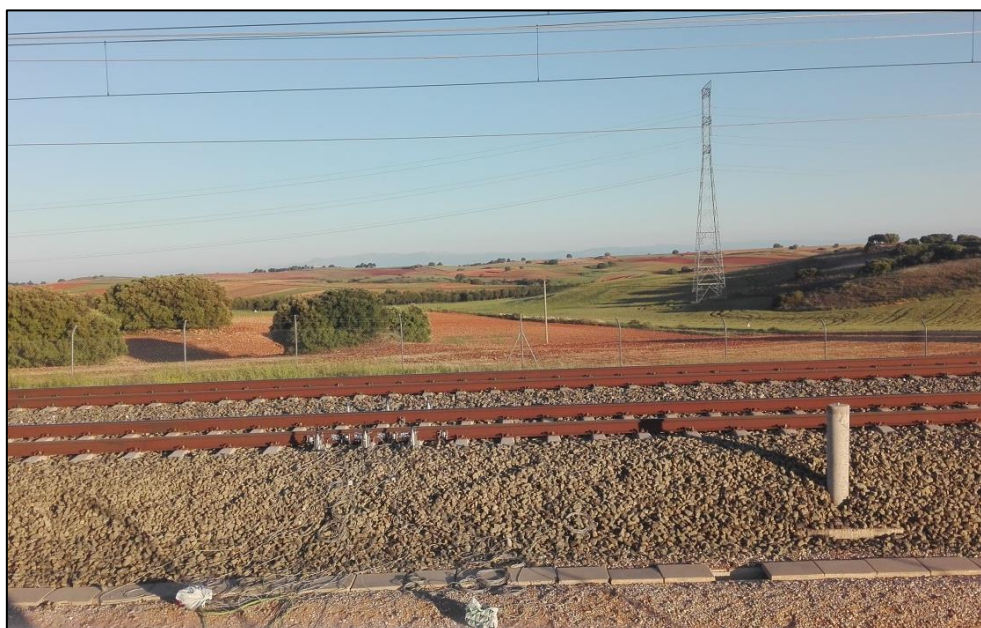
FIGURE 4: PK 74+233 MADRID-BARCELONA HIGH SPEED LINE- STRAIGHT TRACK SECTION
