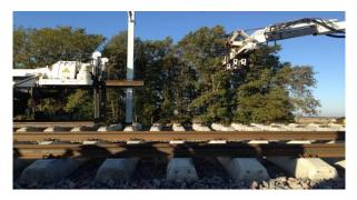
Innovations in laying long welded rails in construction of new high speed lines in France reducing time and costs by factor 2 against traditional methods
